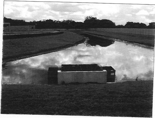
Drainage Pond and Control Structure
