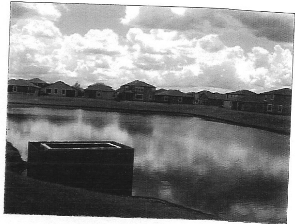
Drainage Pond and Control Structure
